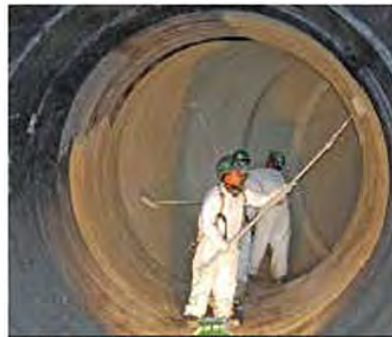
Top coating of CFRP in a large-diameter PCCP
