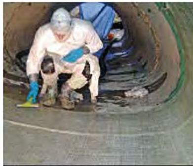
Repair of joints in oval-shaped concrete culvert
