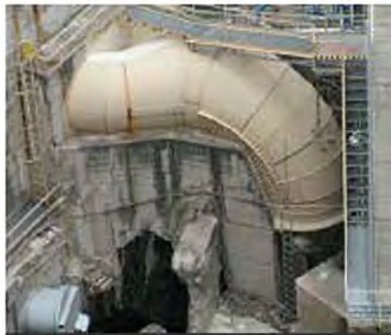
90-year old riveted steel penstock with challenging geometry repaired with CFRP
