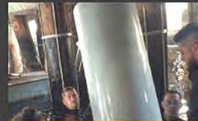
PileMedic® jacket installed prior to placement of grout
