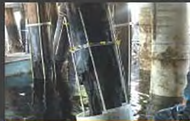
Spacers and FRP rebar attached to the pile
