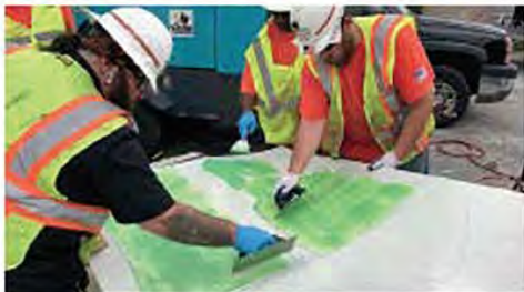
SuperLaminate™ was installed to bridge a gap
