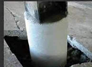
Section after strengthening with PileMedic®
