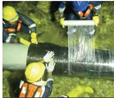
External repair of oil pipe submerged in water using QuakeWrap
